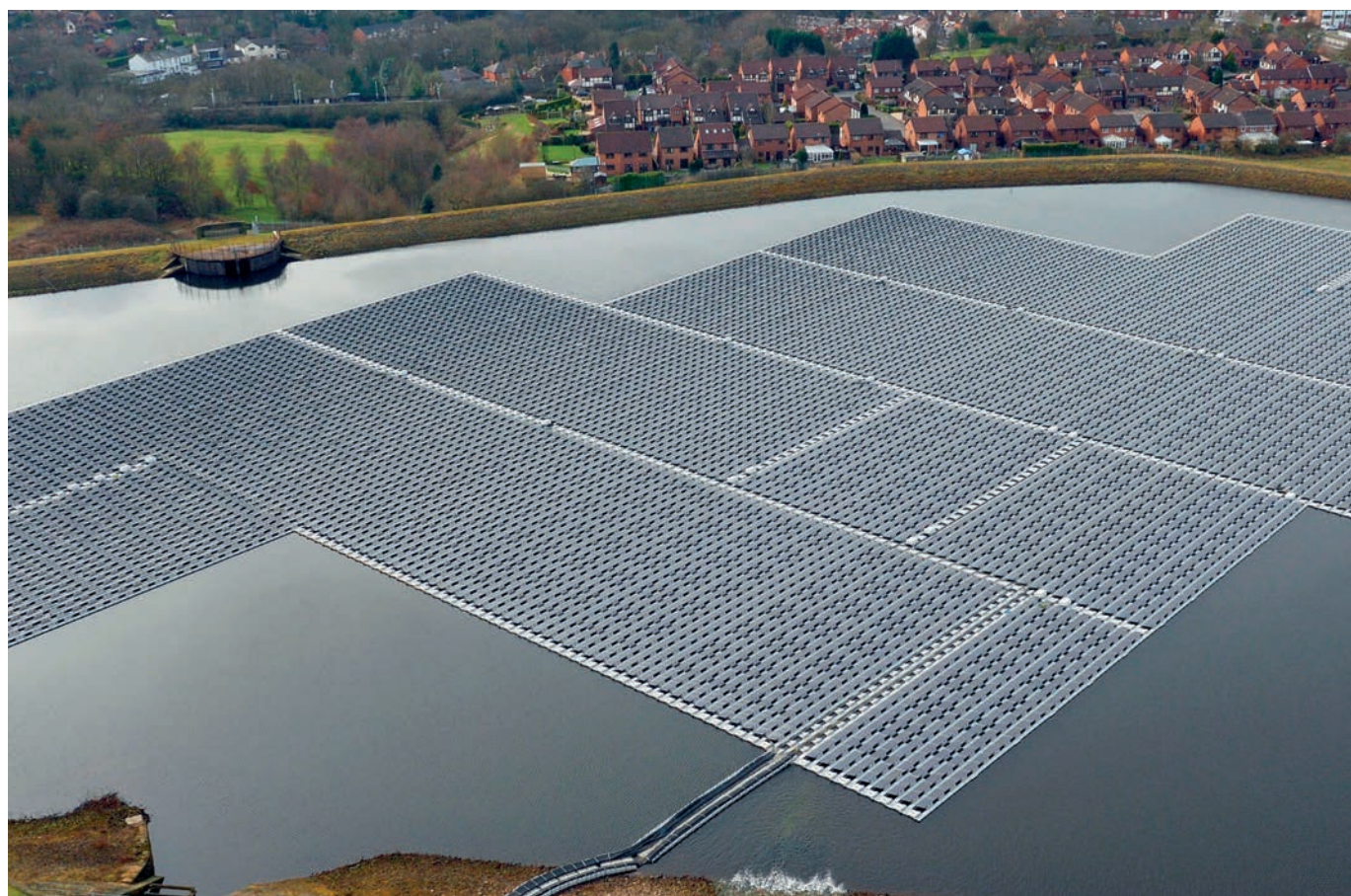
Pictured: Floating solar panel facility at Godley reservoir, East Manchester
