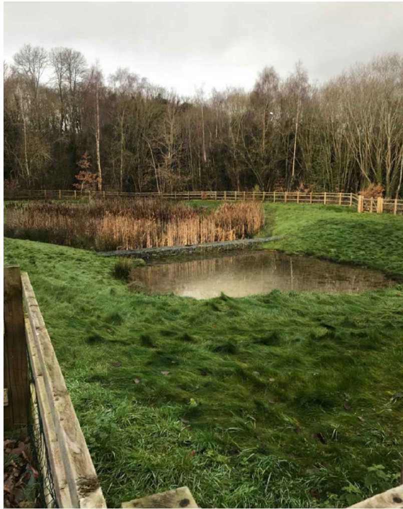
PHOTO OF CONCRETE SEDIMENT FOREBAY
